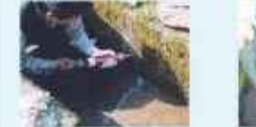
水路のひび割れ補修<br>
